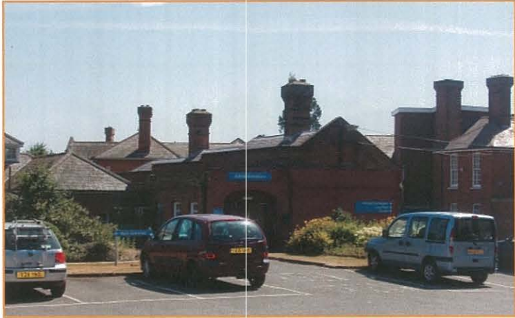
Figure 11 Example of the building heights and the building clutter in the north
