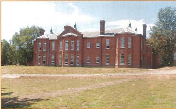
Figure 10 Post-graduate Centre building on the south east corner of the old building structure
