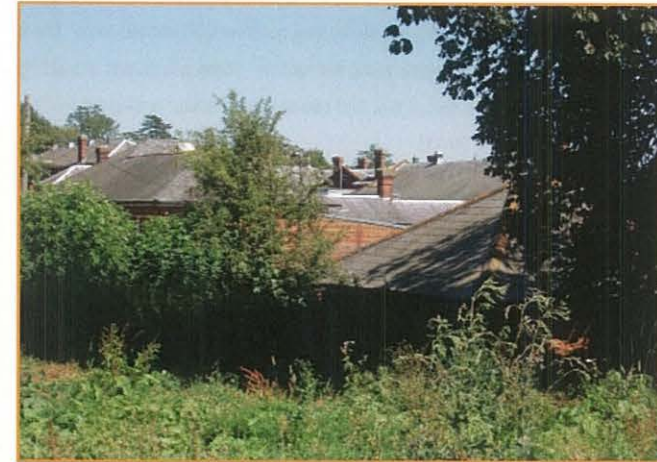
Figure 8 Example of building levels in the west of the site and the buildings cut into the slope
