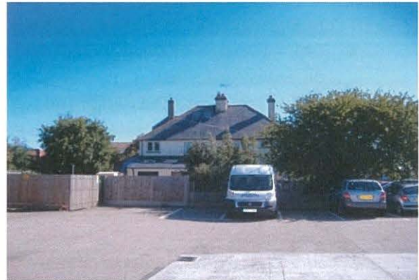
Rear elevation of 3 and 5 Pier Avenue
